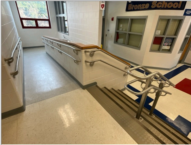
ACCESSIBLE INTERIOR RAMP
