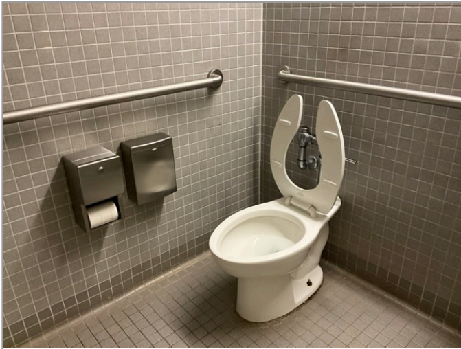
TOILET STALL OVERVIEW
