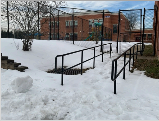
ACCESSIBLE ROUTE TO PLAYGROUND
